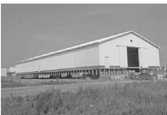
Need to move or hold up a barn, pole barn, silo, house, or anything over size or weight? We have the equipment, personnel, experience & insurance. (616) 836-1911
